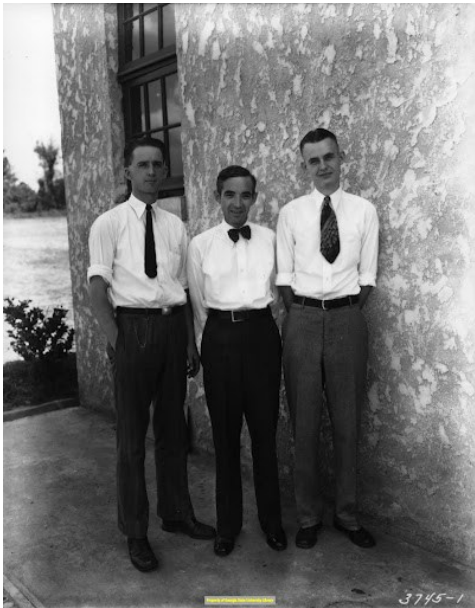
Three engineers stand next to the transmitter building at WSB's East Lake antenna tower. The man in the middle is A.W. Shropshire, circa 1930. WSB Radio Records, Popular Music and Culture Collection, Special Collections and Archives, Georgia State University Library.
