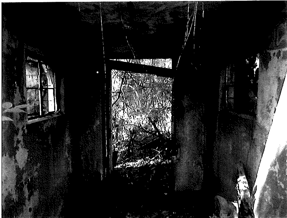
Photo 29: Milking barn (B5), interior door of western room; looking west.
