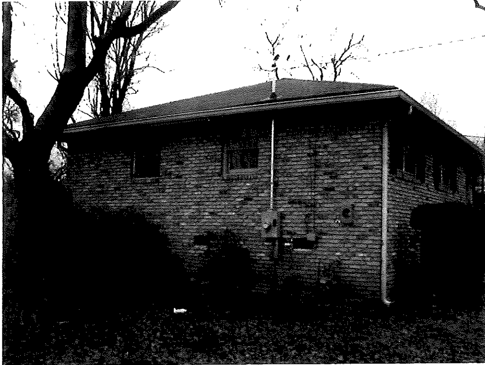
Photo 2: West elevation; looking northeast.
