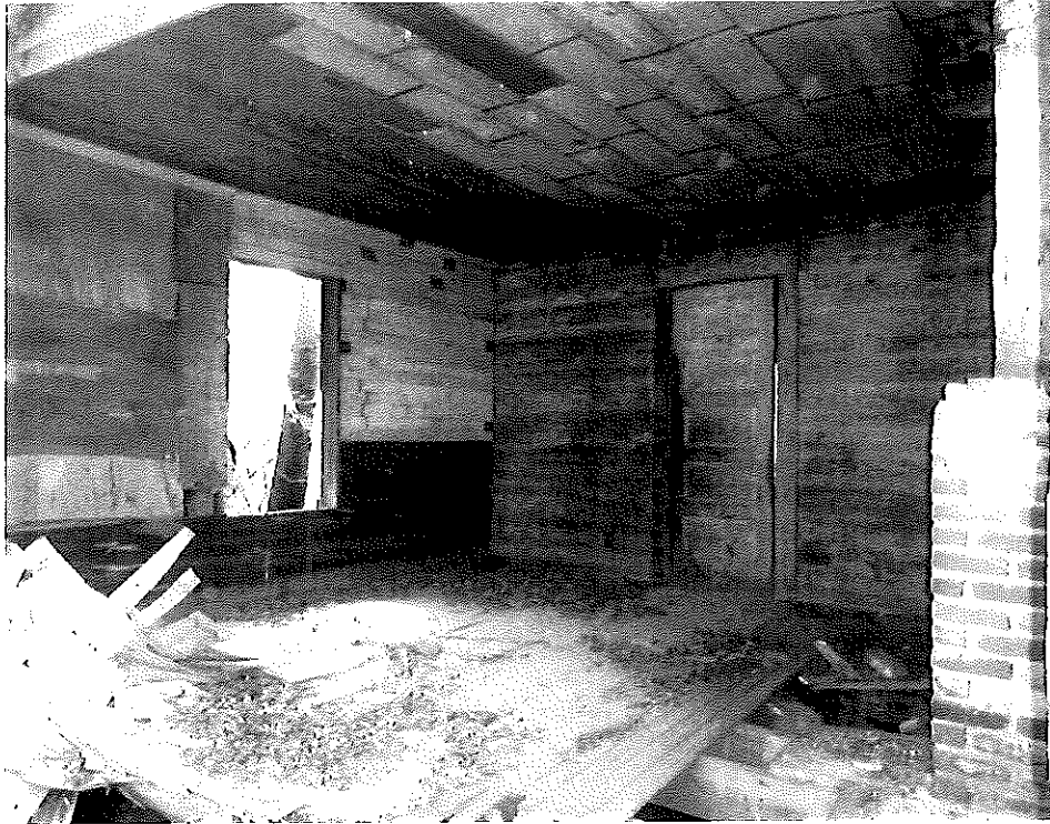
Photo 12: Tenant house (B2) interior room; looking north.
