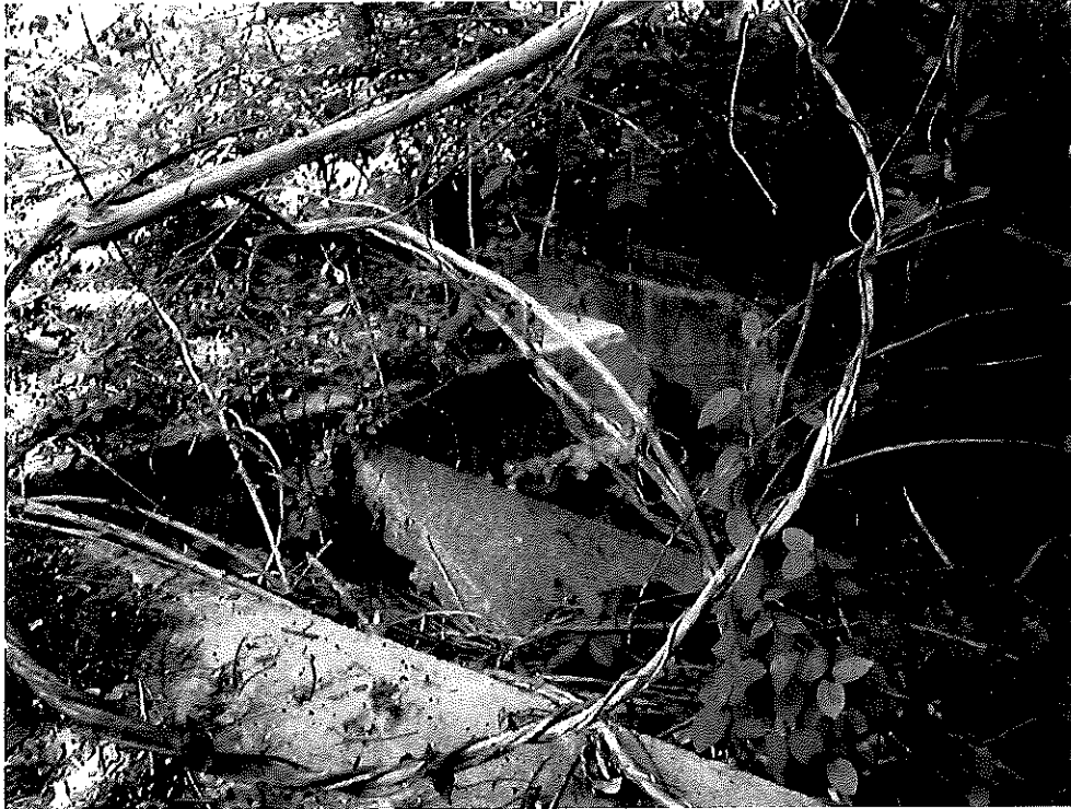
Photo 32: Milking barn (B5), exterior drain from stanchion room and culvert; looking south.
