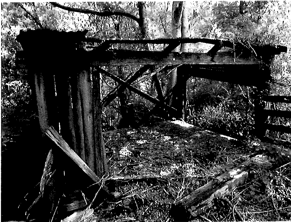
Photo 31: Milking barn (B5), northern cattle shelter; looking north.
