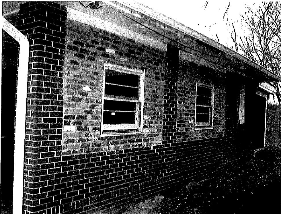
Photo 5: East elevation; looking northwest.
