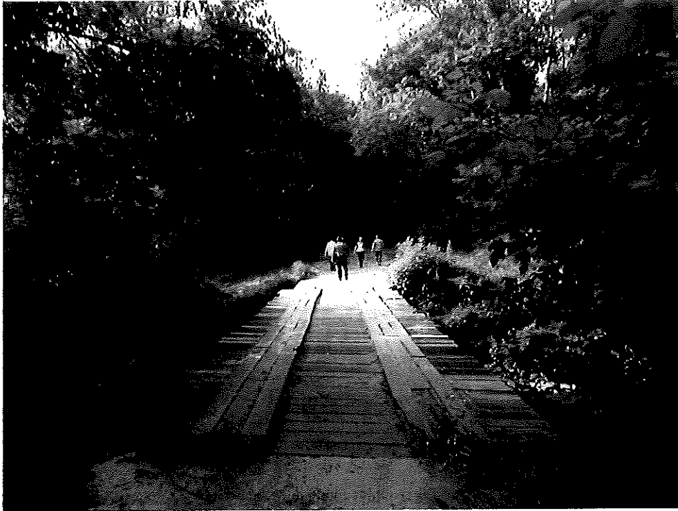
Photo 6: Bridge over South River, erected by C.H. Smith (north approach); looking south.
