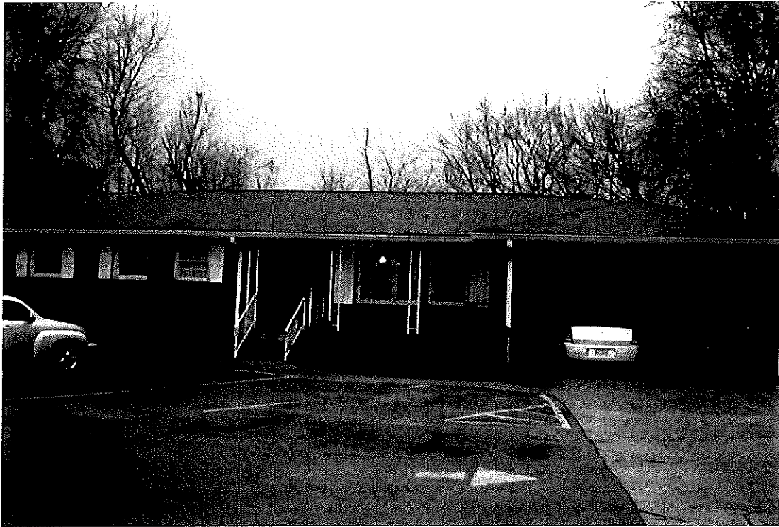
Photo 1: Front (south) elevation; looking north.
