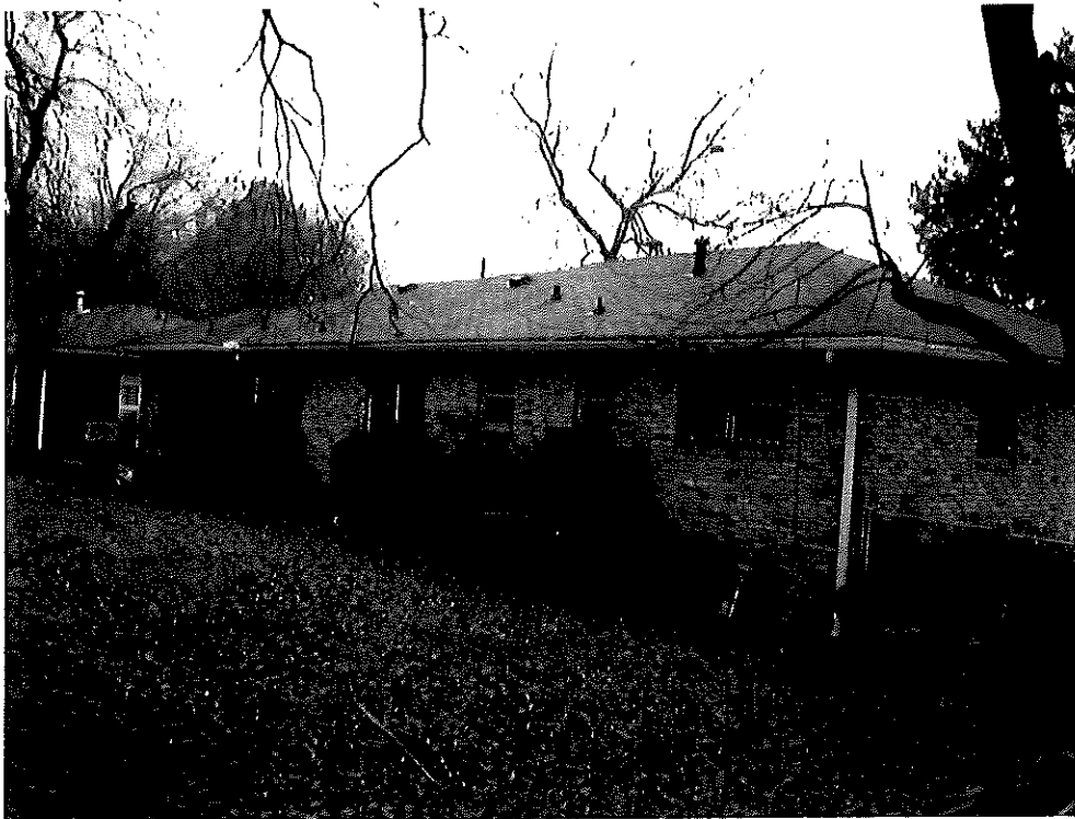
Photo 3: Rear (north) elevation; looking southeast.
