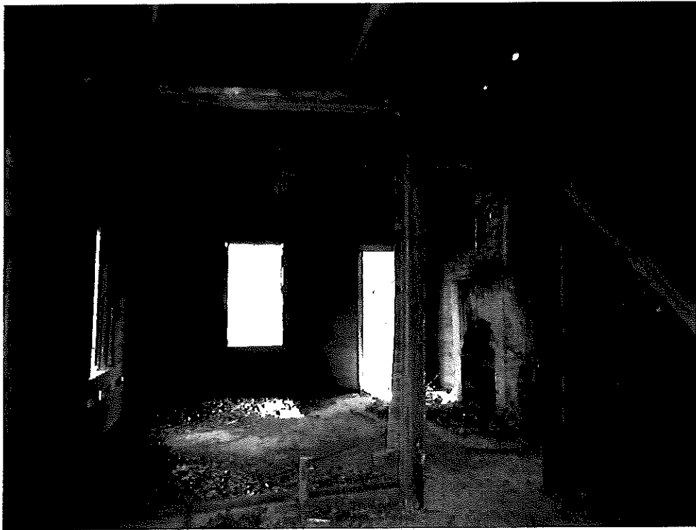
Photo 9: Tenant house (B1) interior; looking east.
