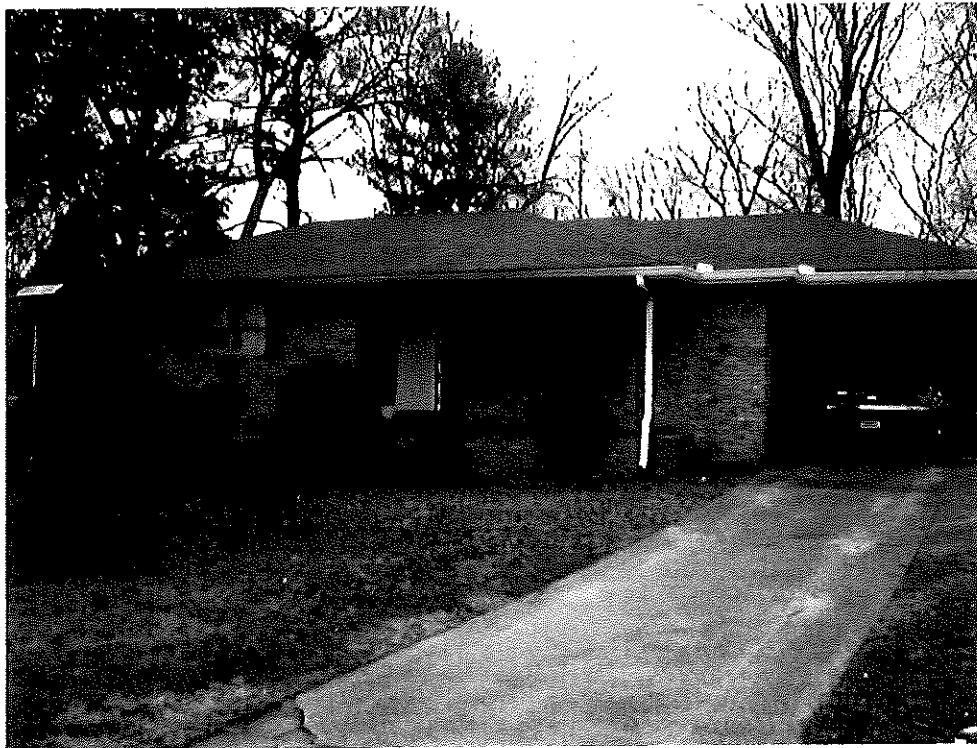
Photo 1: Front (south) elevation; looking northwest.
