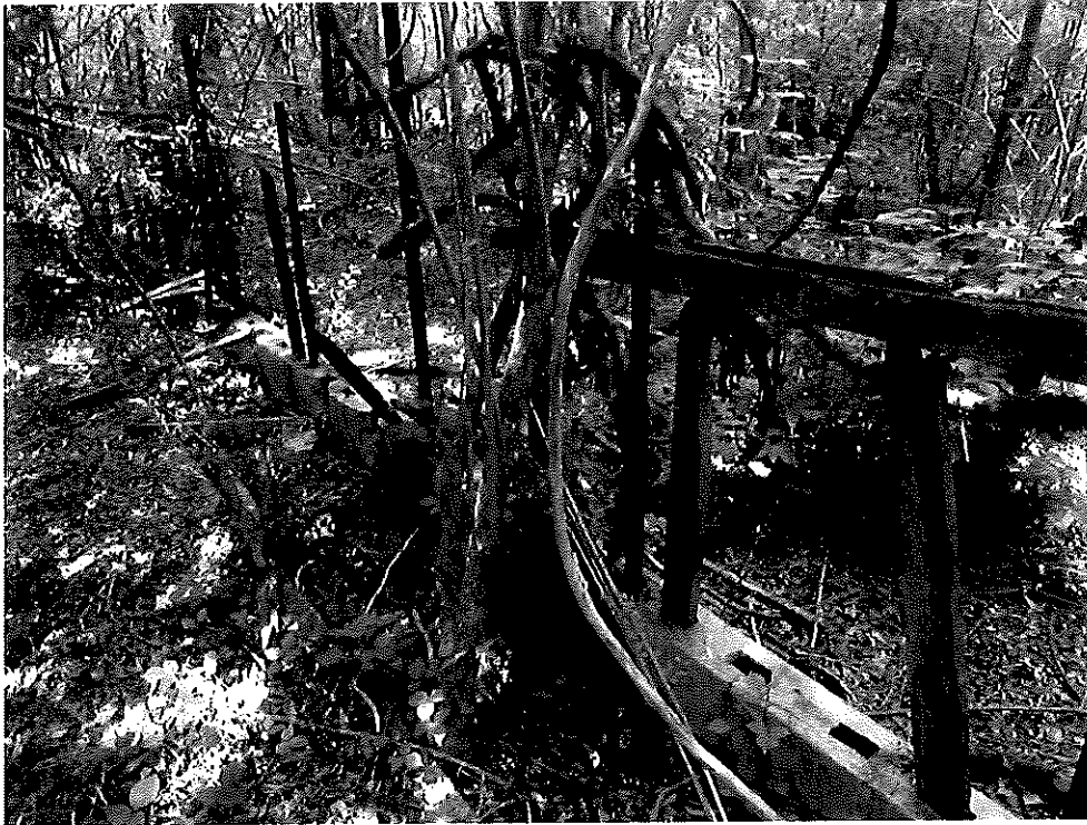
Photo 30: Interior of milking barn (B5), cattle stanchion remnants and drains; looking southeast.
