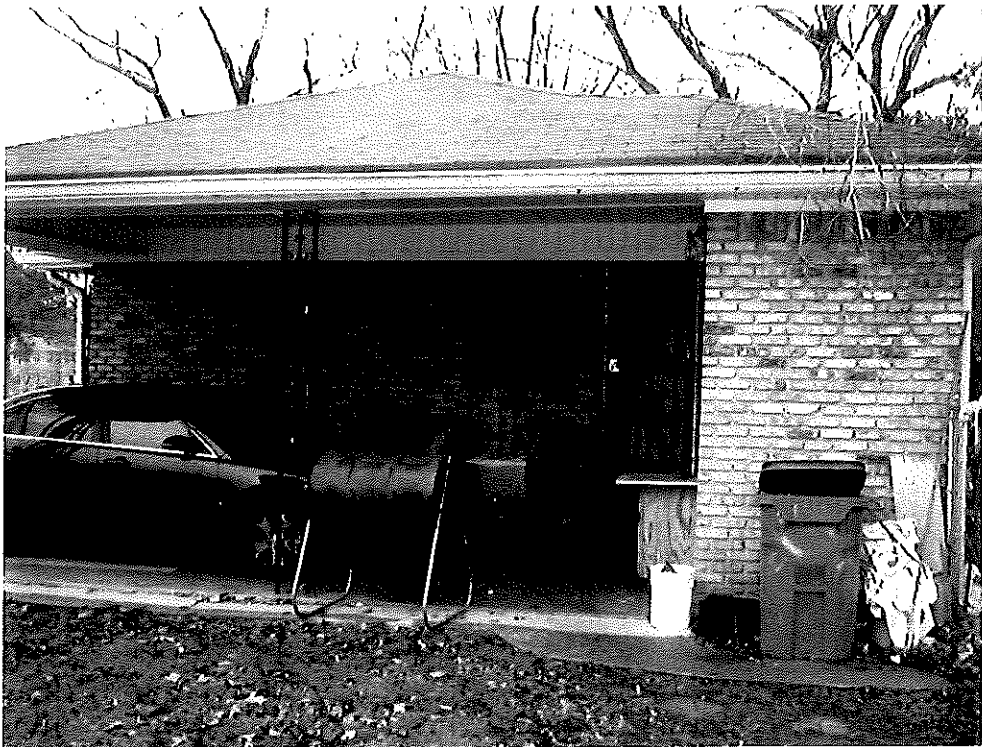
Photo 5: East elevation; looking west.
