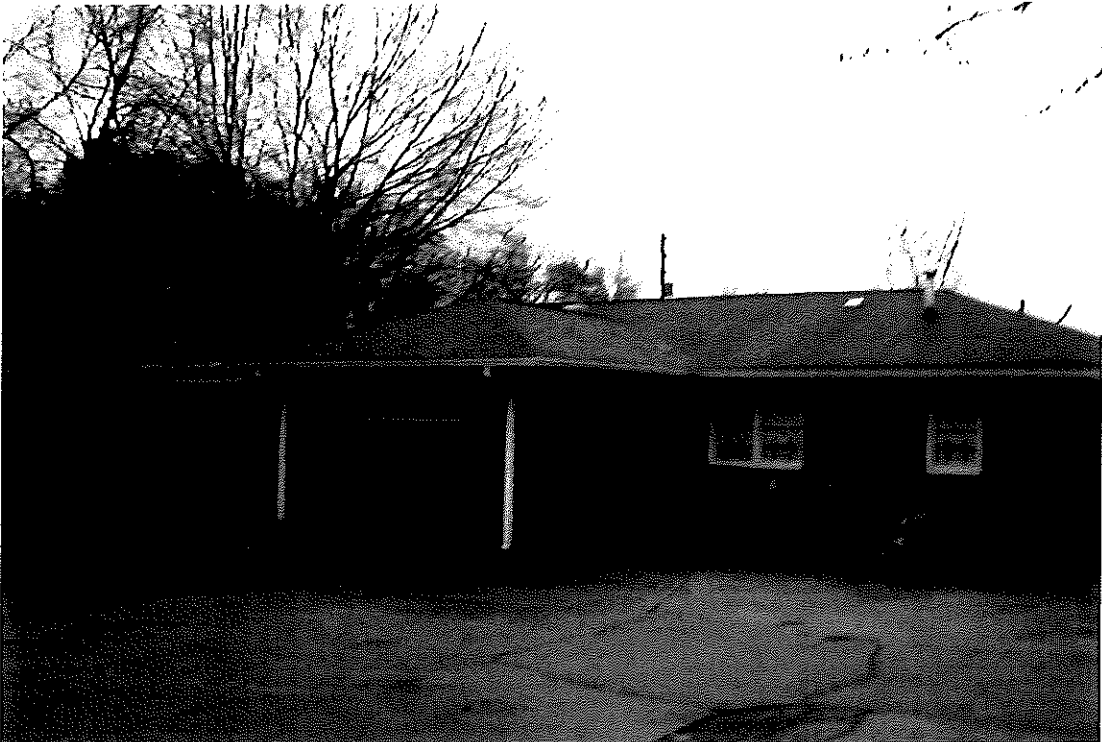
Photo 3: Rear (north) elevation; looking southeast.
