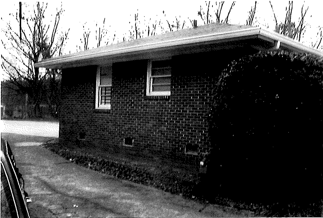
Photo 2: West elevation; looking northeast.
