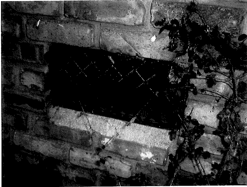
Photo 6: Craw space grate (west elevation); looking east..
