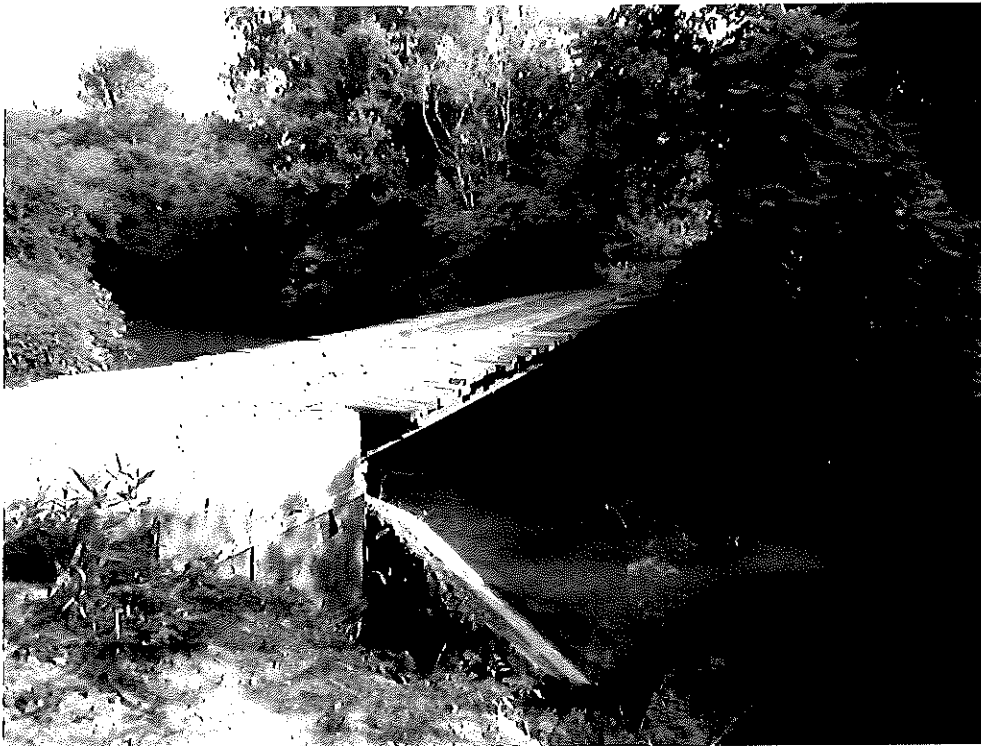
Photo 7: Bridge over South River, east span; looking northwest.
