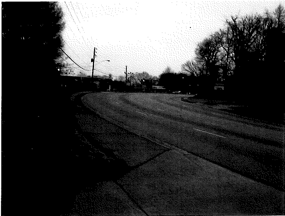
Photo 9: Right-of-way; looking east.
