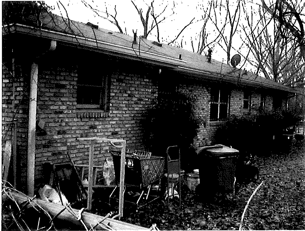
Photo 4: Rear (north) elevation; looking southwest.
