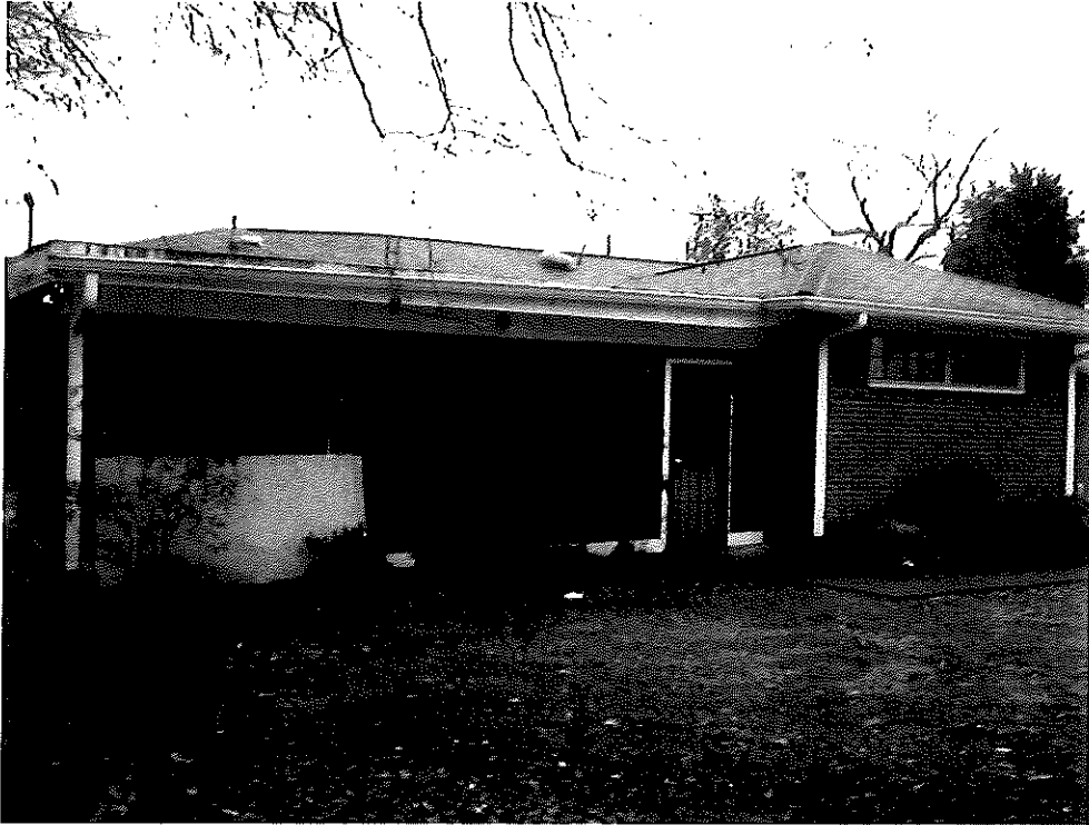
Photo 4: Rear (north) elevation; looking southwest.
