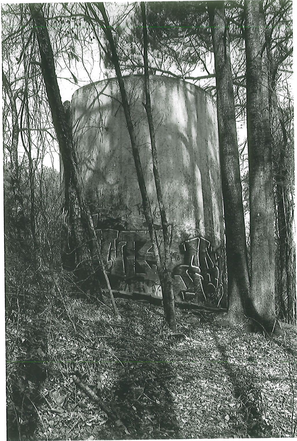
Decatur Waterworks DeKalb County, Georgia Photograph | 9 of 33
