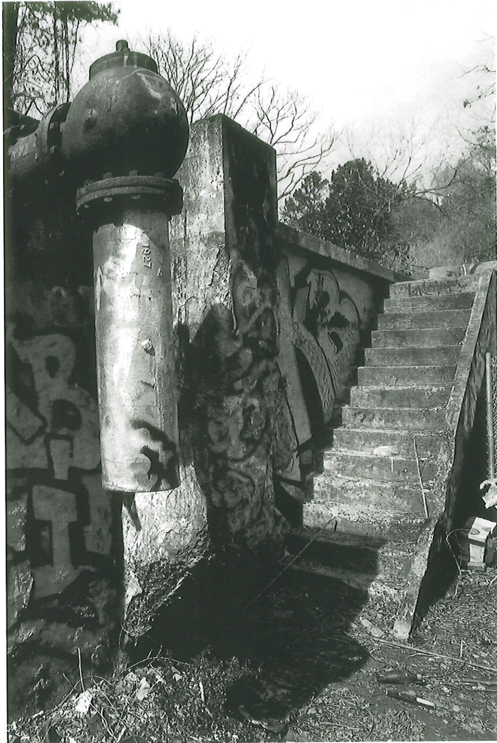
Decatur Waterworks DeKalb County, Georgia Photograph 9 of 33
