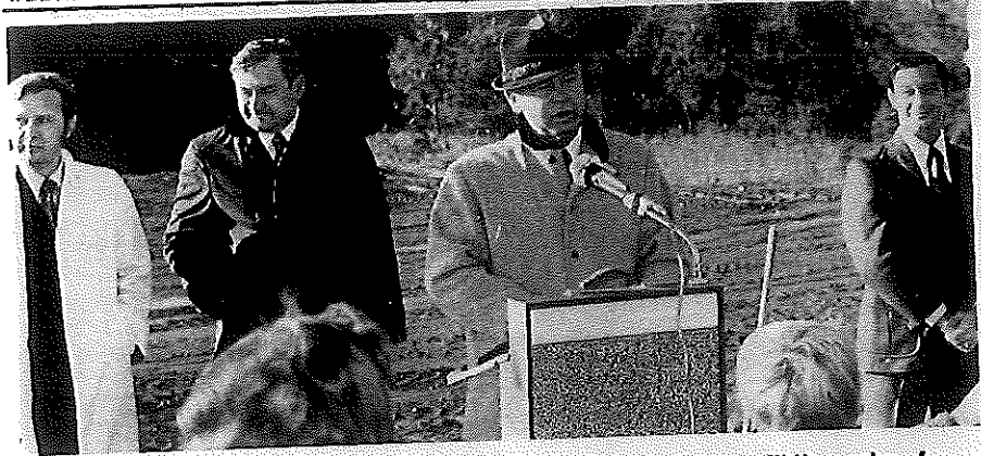
NEW DUNWOODY AREA SCHOOL UNDERWAY--(Background) Rodney Wells, member of DeKalb Board of Education, Dr. Clyde A. Holsclaw, North Area Assistant Superintendent, and Ronald Stegall, principal of Dunwoody High School, (left to right) along with a large turnout of Dunwoody residents, listen to comments by DeKalb School Superintendent, Dr. Jim Cherry, at the groundbreaking ceremony for a DeKalb Elementary School to be located at 1877 Vanderlyn Drive. The ceremony was held last Wednesday, with Dr. Holsclaw presiding. Also participating in the program were Rev. Joe Spain, pastor of North Peachtree Baptist Church; Floyd Kornegay, principal of Kingsley Elementary School; Ronald Stegall; Harold Wells, principal of Dunwoody Elementary School; and the Rev. Owen Kellum, pastor of Dunwoody United Methodist Church.
