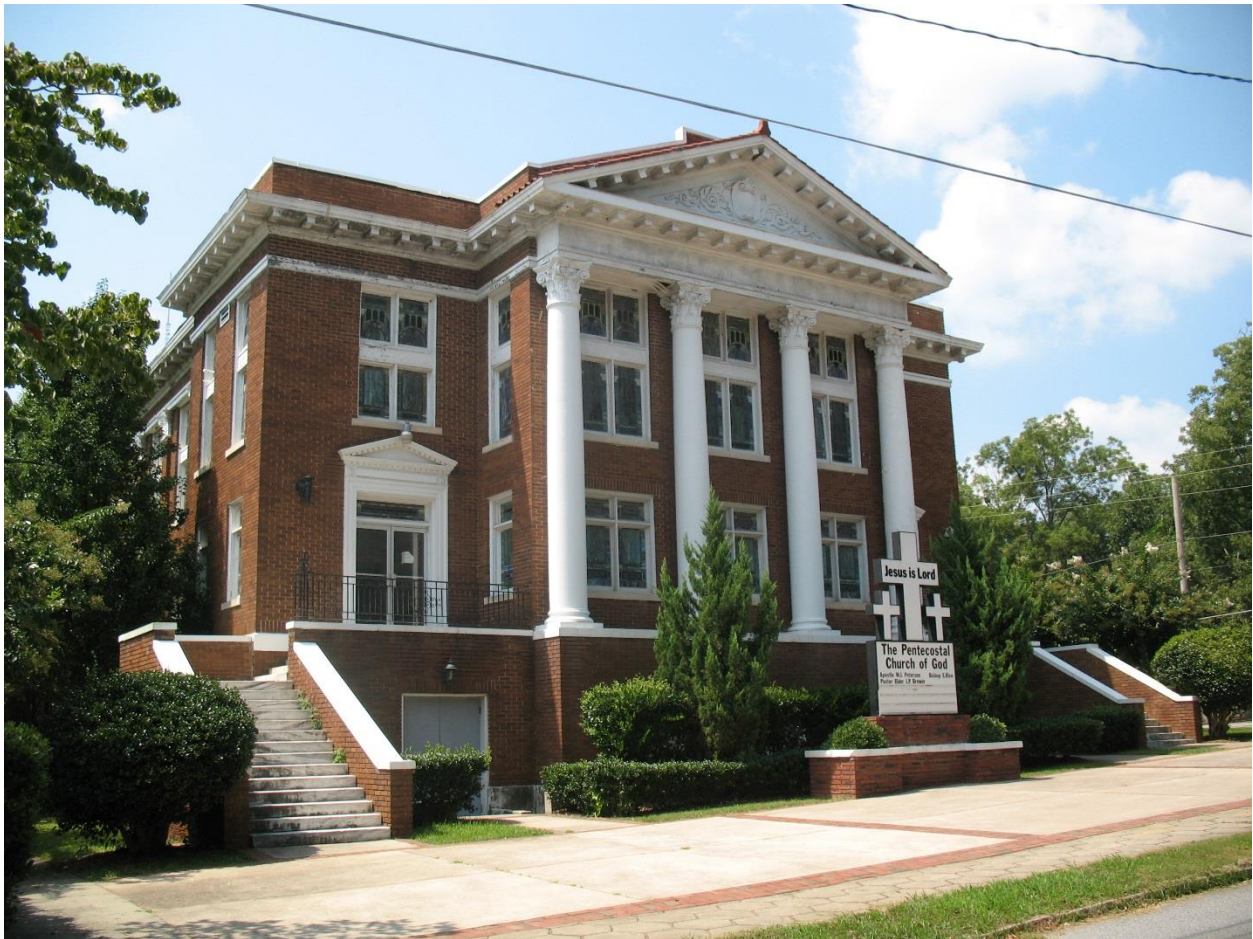
Kirkwood Baptist Church Today's Pentocostal Church of God, 110 Howard Street NE
