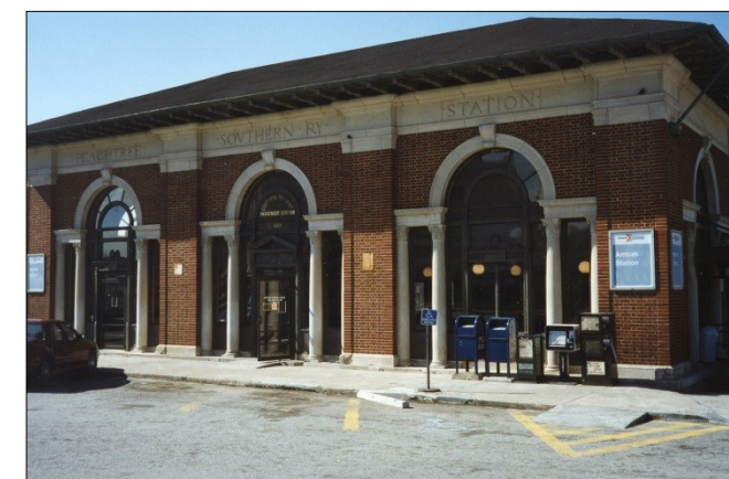
Peachtree Station located on land that once was part of Peachtree Trail.
