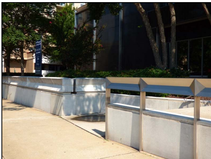
The original concrete and stainless steel railings.
