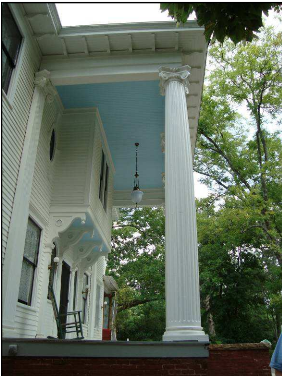
The portico features two-story Ionic columns.
