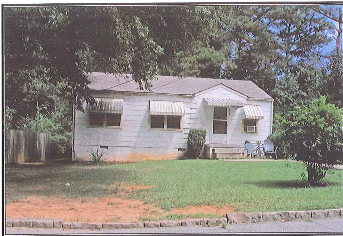
Photograph 11 – Representative view of residence in Happy Valley Subdivision looking east from Deacon Lane.
