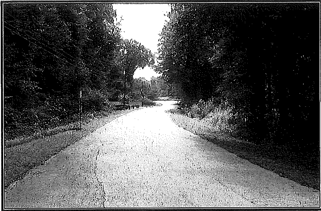
Photograph 5 – Representative streetscape view in Carver Hills Subdivision looking southwest along N. Carver Drive (North side of I-285)
