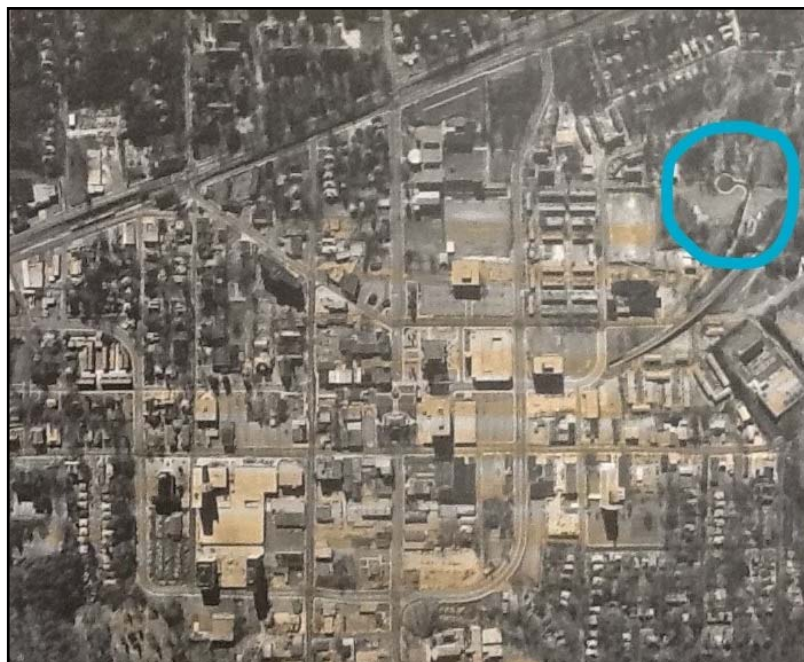
From the DeKalb History Center's photograph collection, a view of downtown Decatur in 1981. The blue circle shows the location of the Swanton Hill Townhomes.
