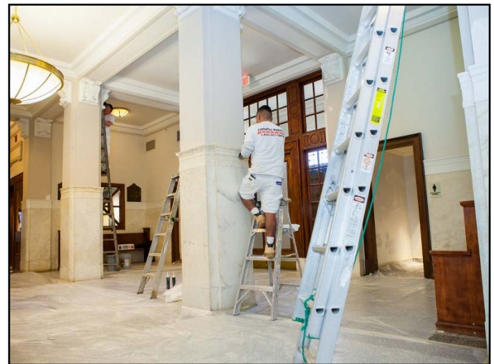
CertaPro team member painting columns in the lobby.
