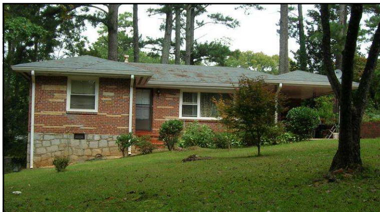
A typical ranch house in DeKalb County, this one is in Belvedere Park.
